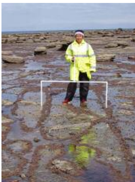
Fig.2 One of a number of narrower rutways identified during the survey
