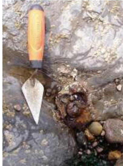
Fig.3 Small iron plate bolted into the bedrock
